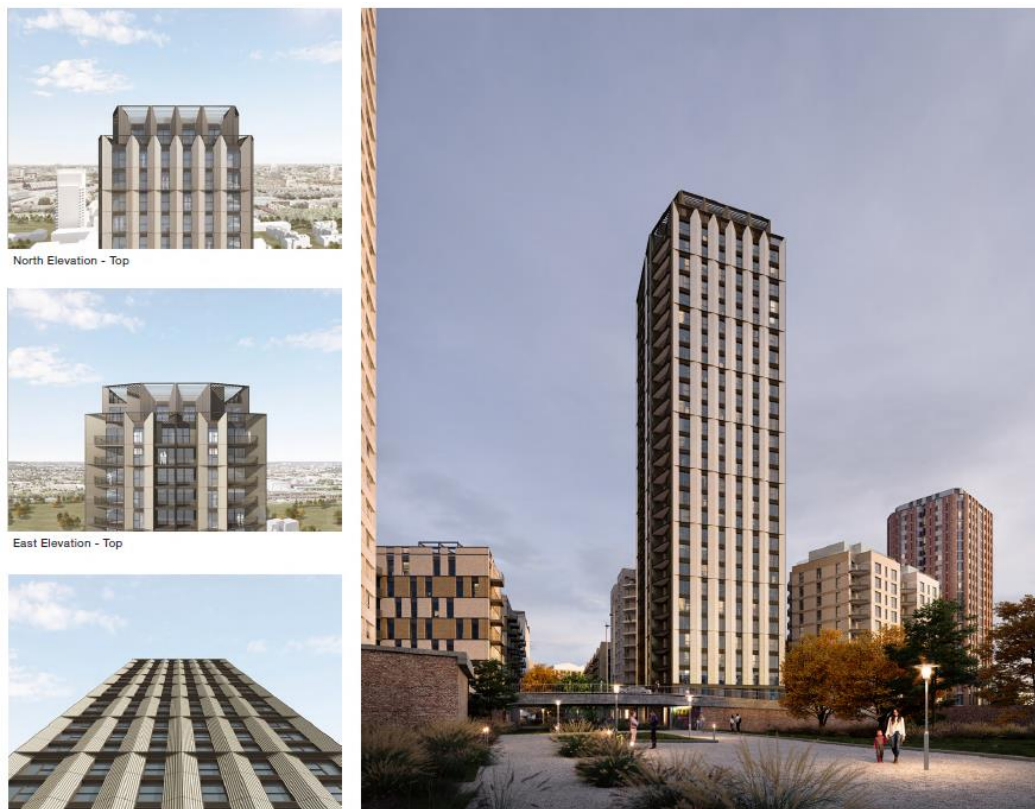
Image 5: North elevation of 5C Waterline Tower
