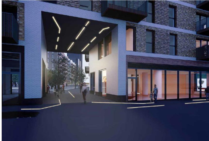
Image 10: Buildings 3C underpass from Dragoon Road
